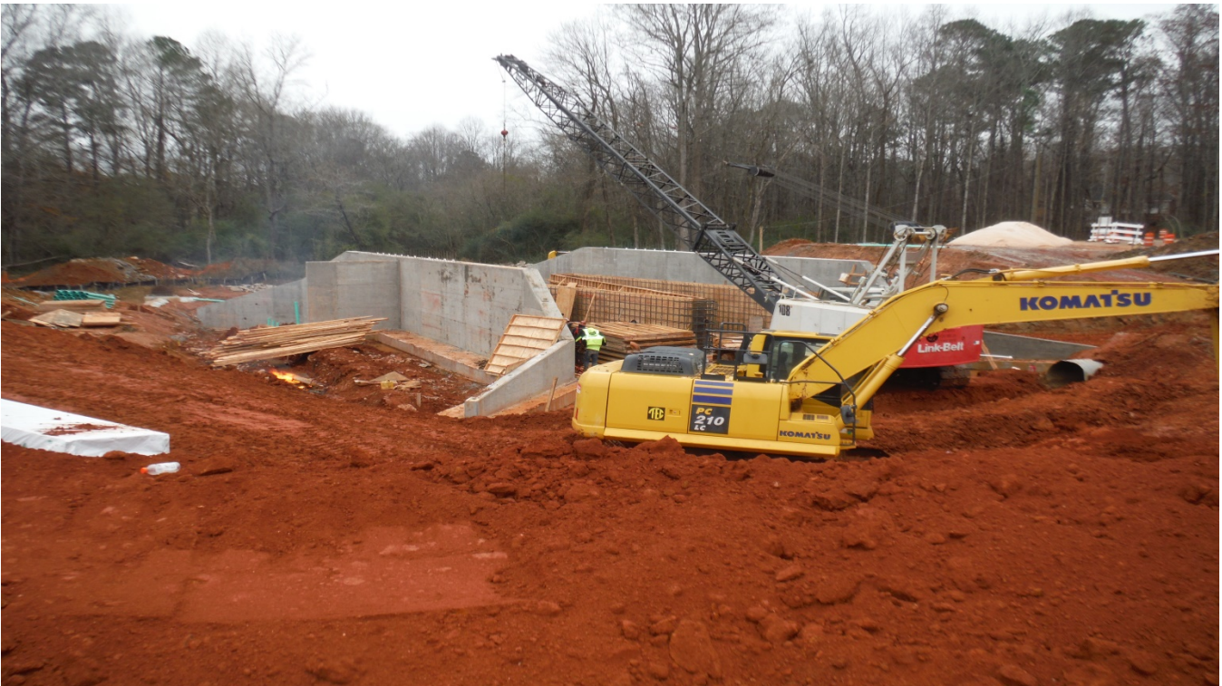
Photo 2: Both walls have been poured. (12/7/17)
