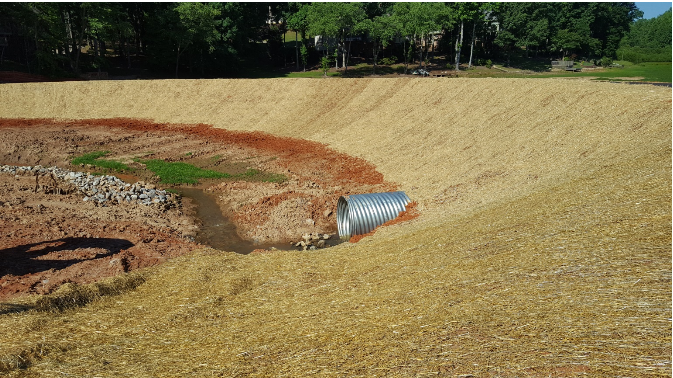
Photo 2: Temporary cofferdam and road detour following temporary stabilization. The metal pipe is part of the dewatering system to be used during construction of the new spillway.
