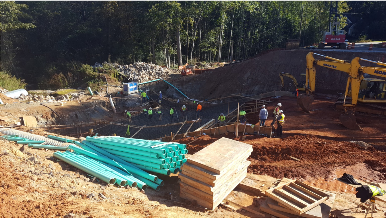
Photo 1: Framing of the spillway on downstream side of the dam. (10/24/17)
