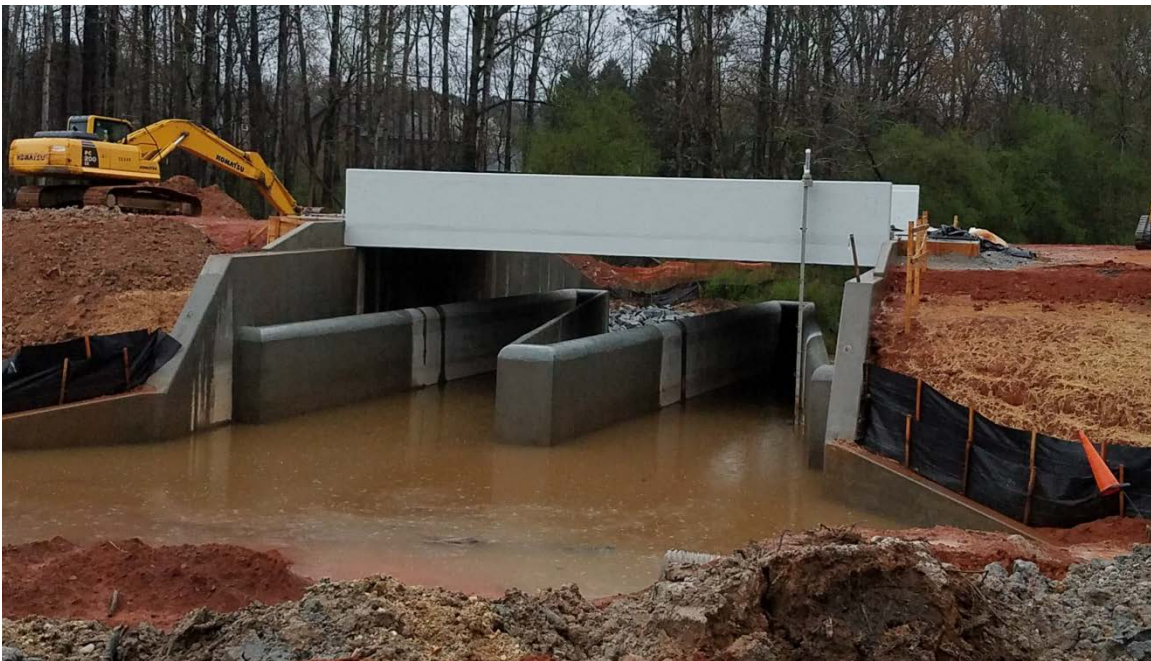
Photo 2: Bridge construction over new spillway. (02/26/2018)
