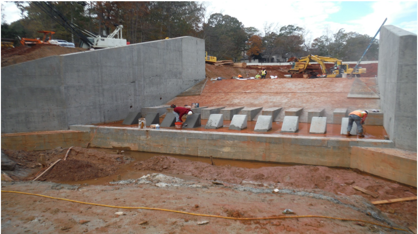
Photo 2: View of Emerald Lake Dam spillway. This is the downstream side of the dam and a view of the energy dissipaters.
