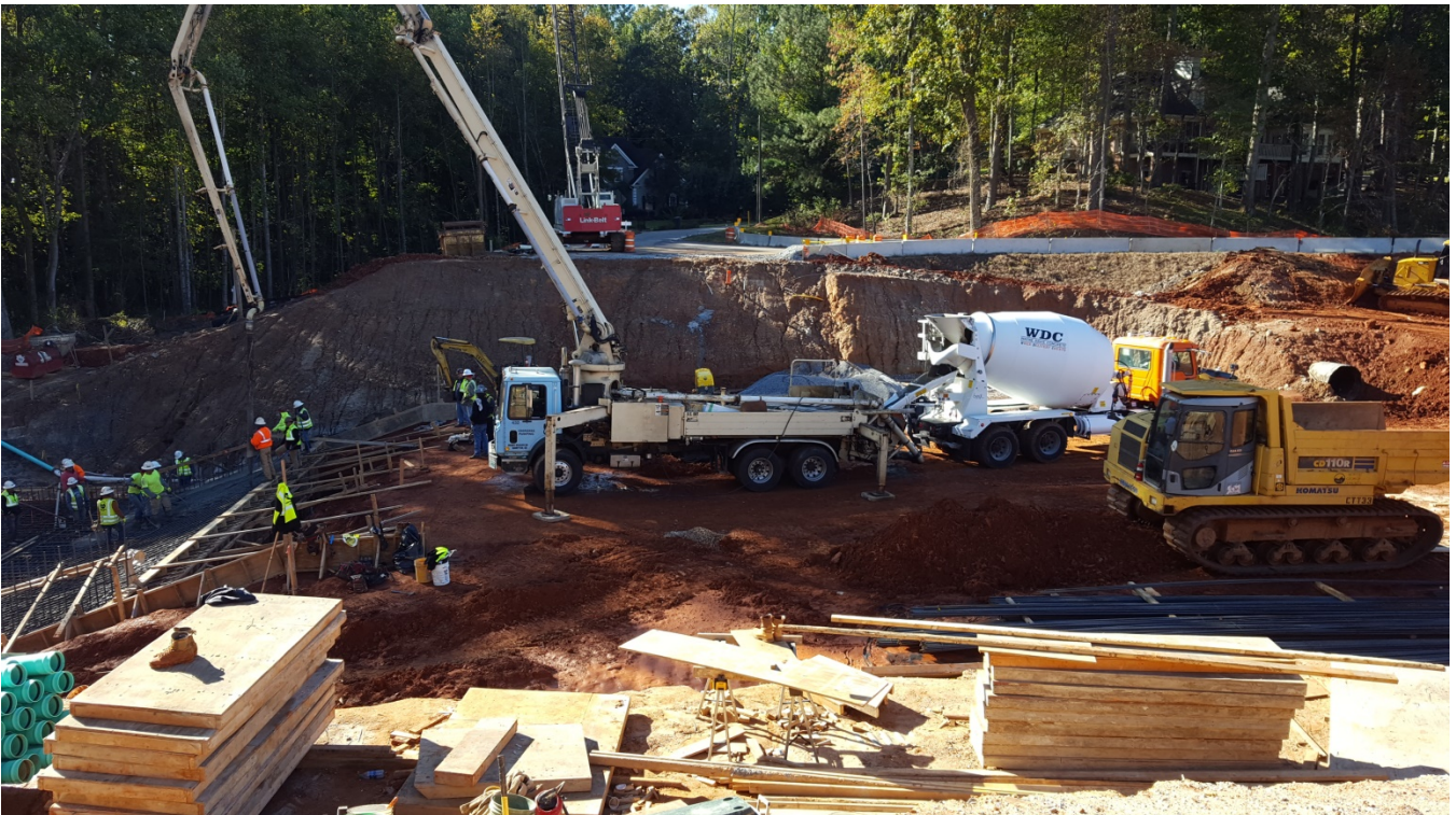
Photo 2: Concrete pouring of spillway on downstream side of the dam. (10/26/17)
