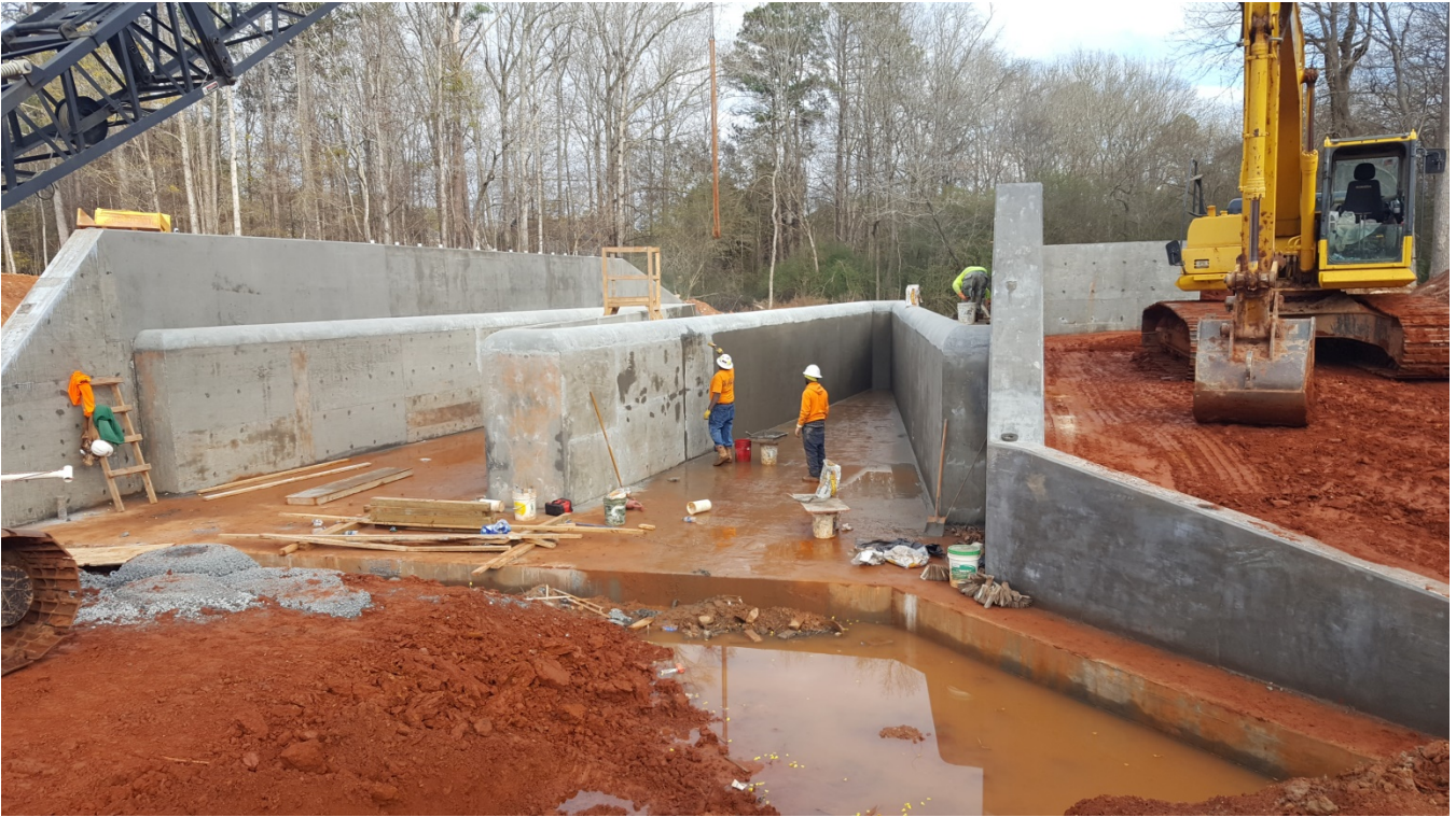
Photo 1: View of Emerald Lake Dam spillway. This view is looking downstream.
