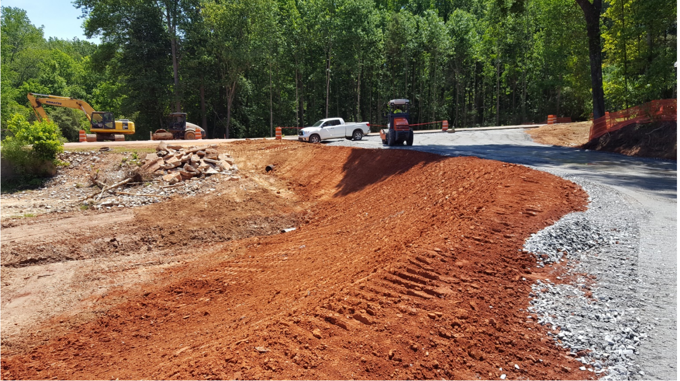
Photo 1: Construction of road detour. (May)
