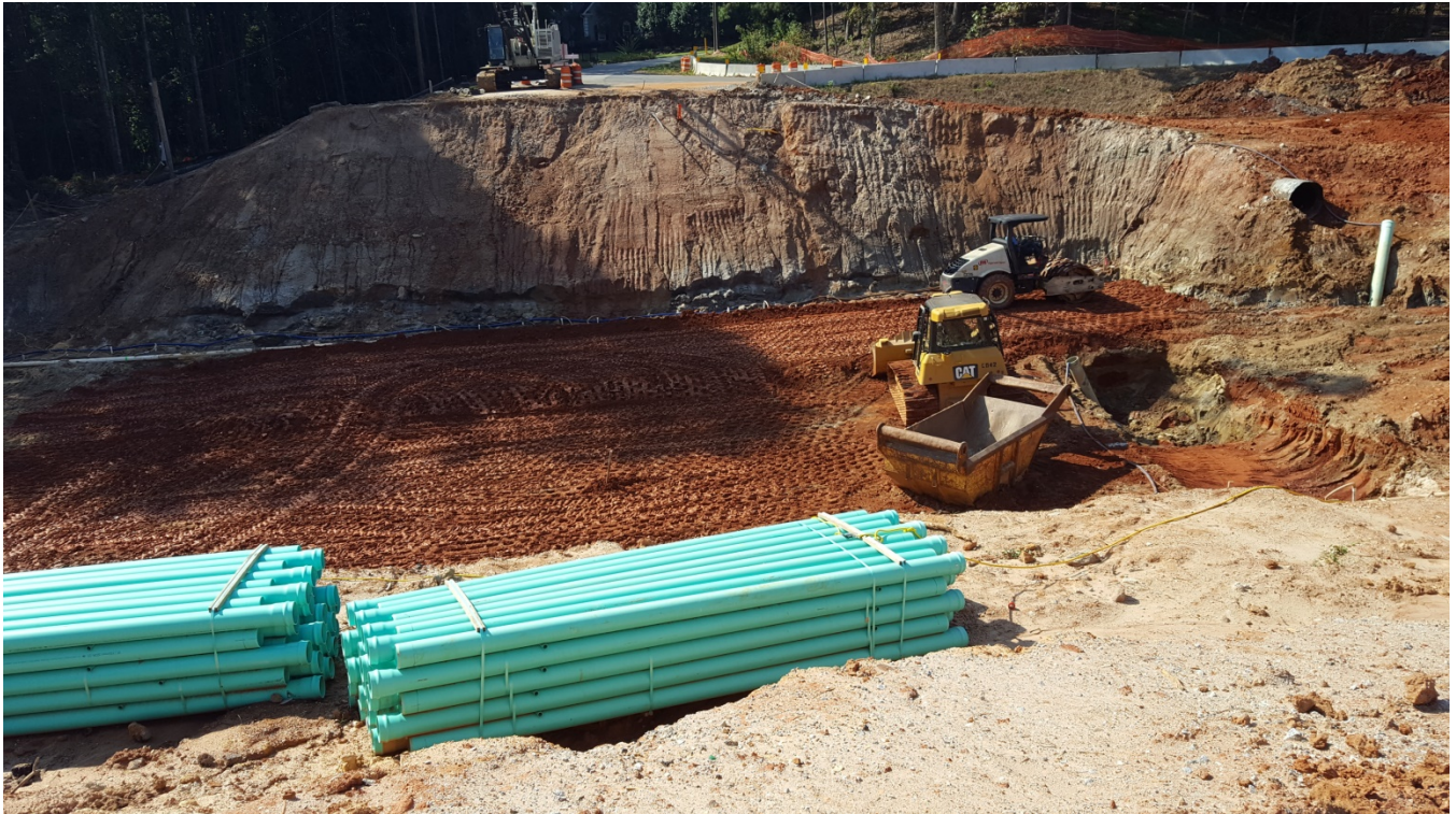
Photo 1: Initial backfilling activities. (9/22/17)
