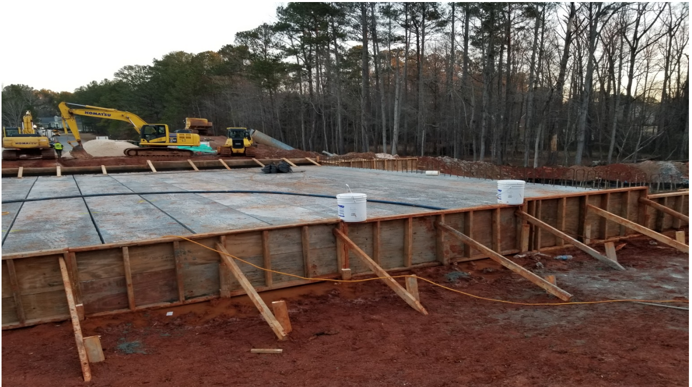
Photo 2: Concrete placement to cover dam spillway. (1/30/18)
