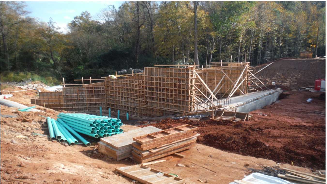
Photo 2: Forming walls to dam spillway.
