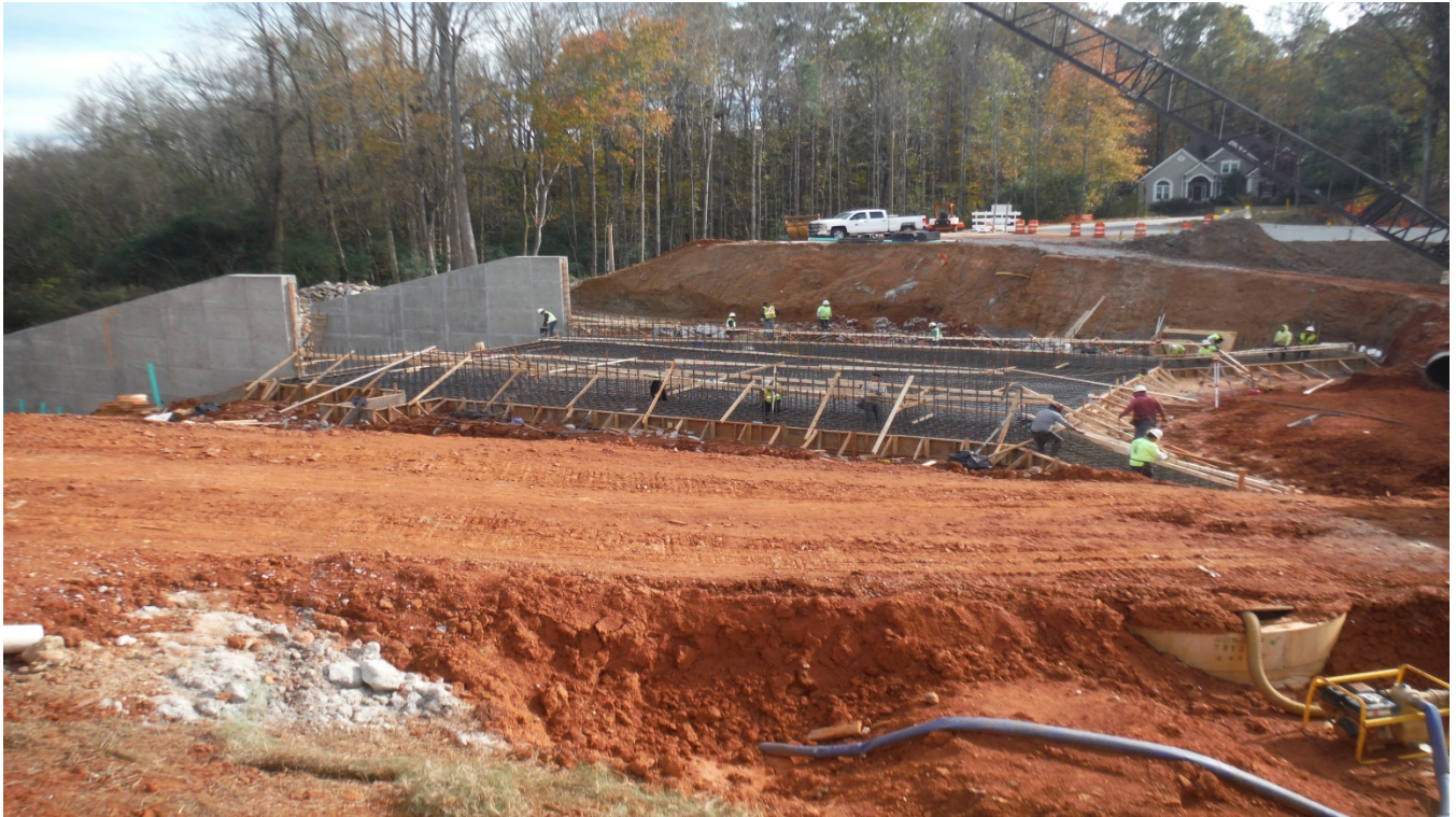
Photo 1: Forming walls for concrete pouring. (11/20/17)
