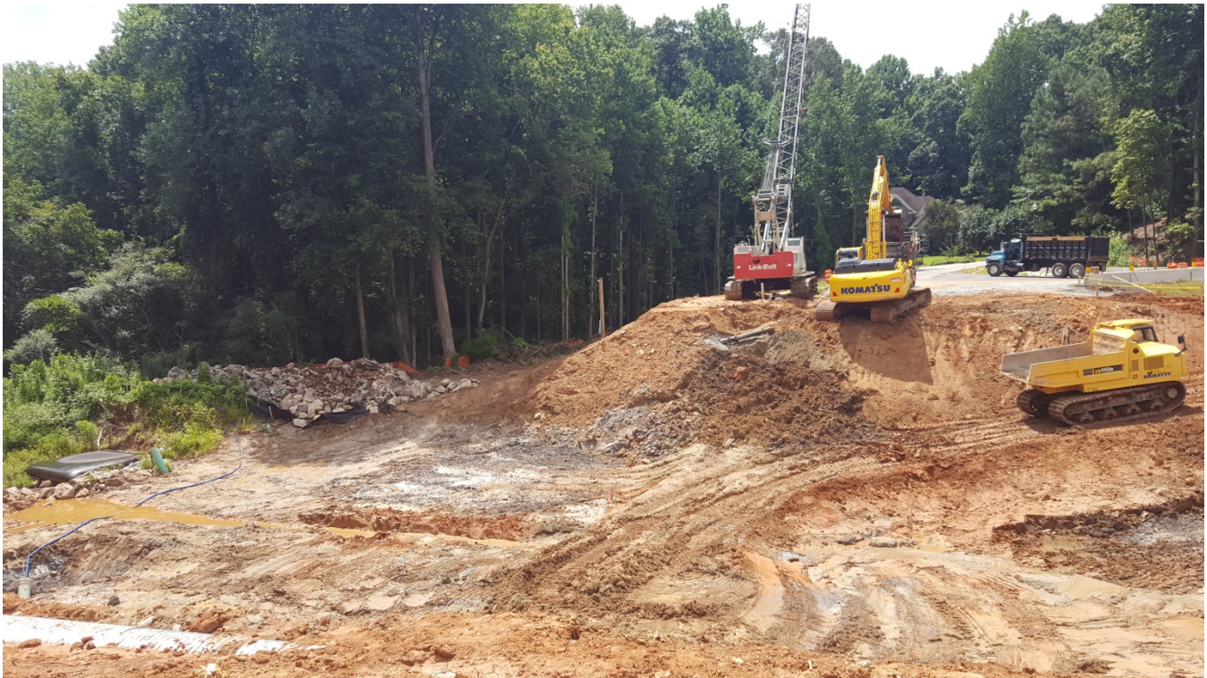
Photo 1: Picture shows location of former road and dam with demolition complete. Dewatering pumps and pipes and diversion pipe are on far left. Contractor is removing bad soils until a solid base is established on which the new dam can be built.
