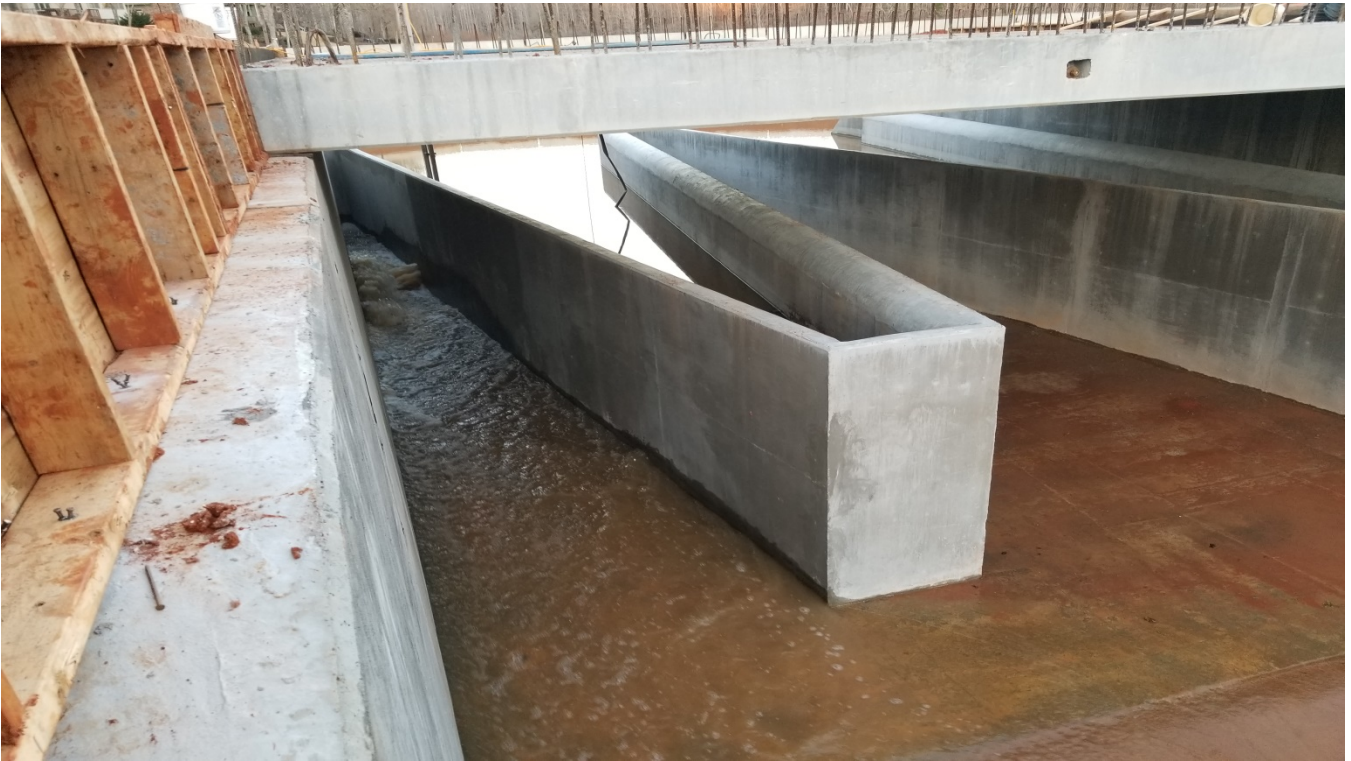
Photo 1: View of water flowing downstream through the newly constructed spillway.
