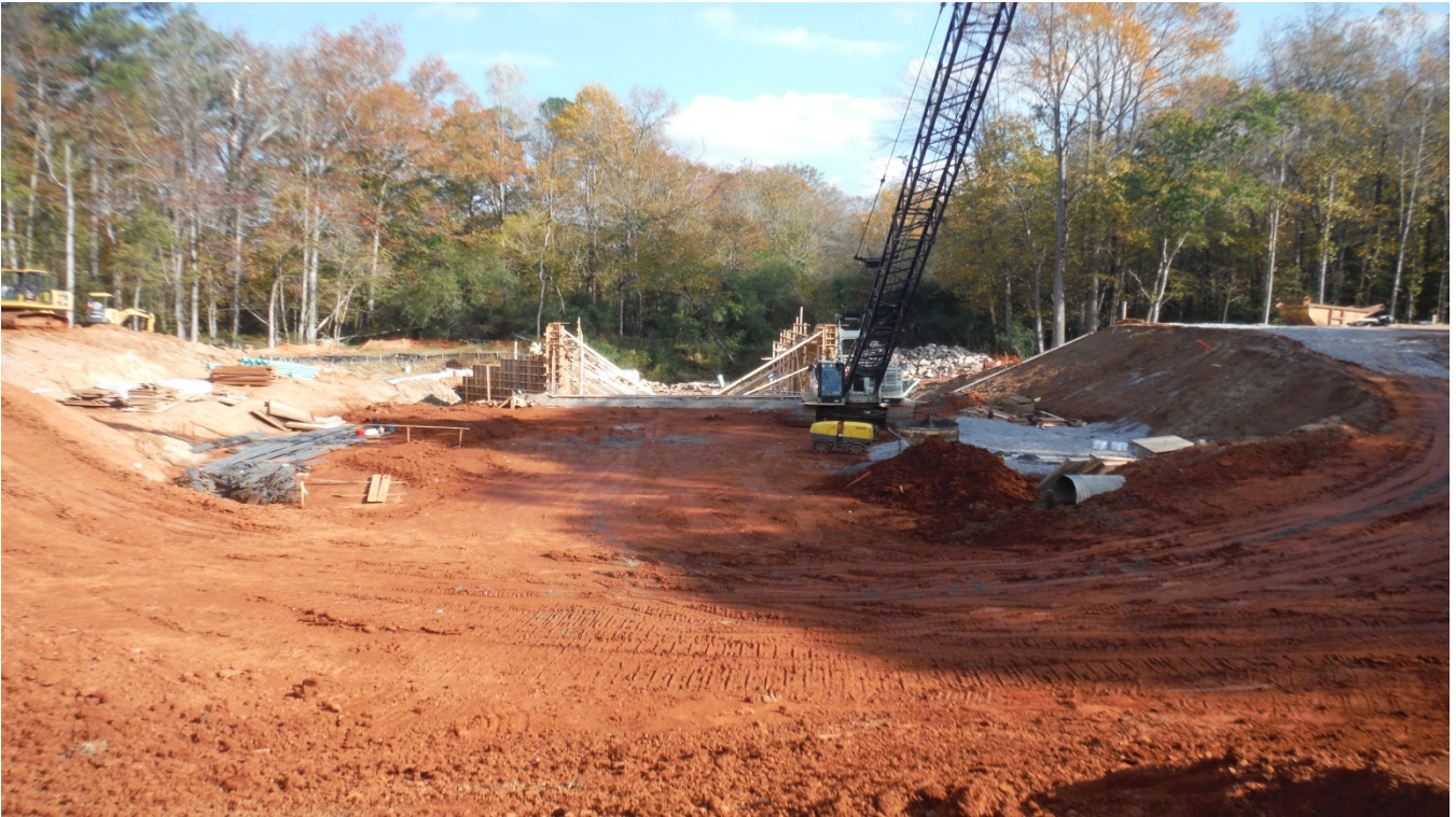
Photo 1: Forming walls to dam spillway (looking downstream).
