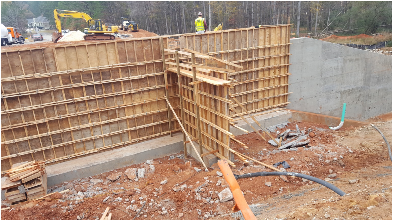
Photo 2: Forming walls for concrete pouring. (11/29/17)
