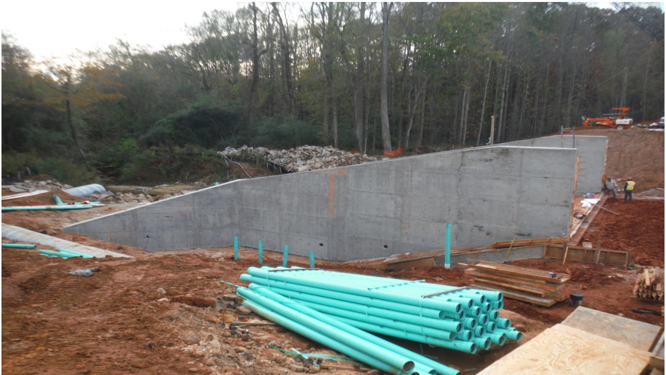
Photo 1: View of Emerald Lake Dam spillway. This is the downstream side of the dam.
