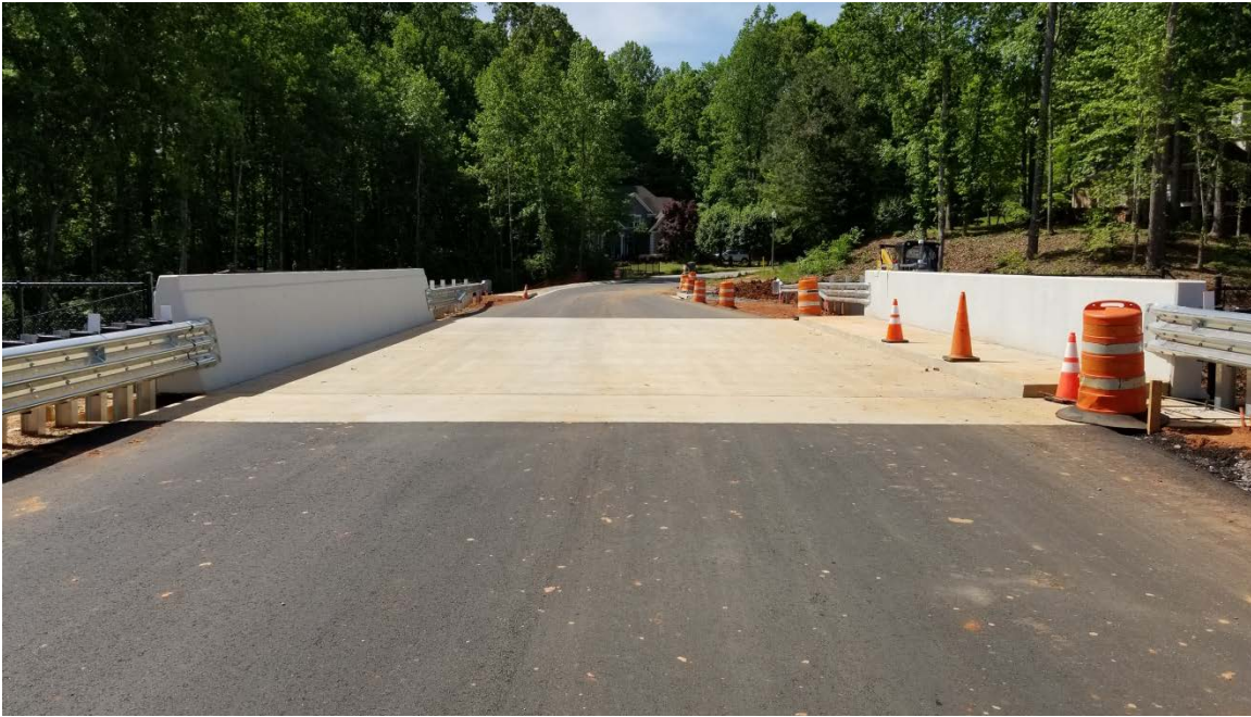
Photo 1: Bridge construction and paving activities over the spillway. (05/03/2018)
